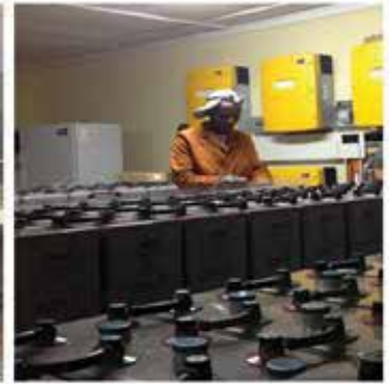
SMA Multiclustor System CAPACITY: 50KW Nairobi
