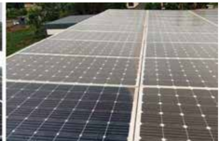
Borehole Solarization CAPACITY: 8 KW Narok
