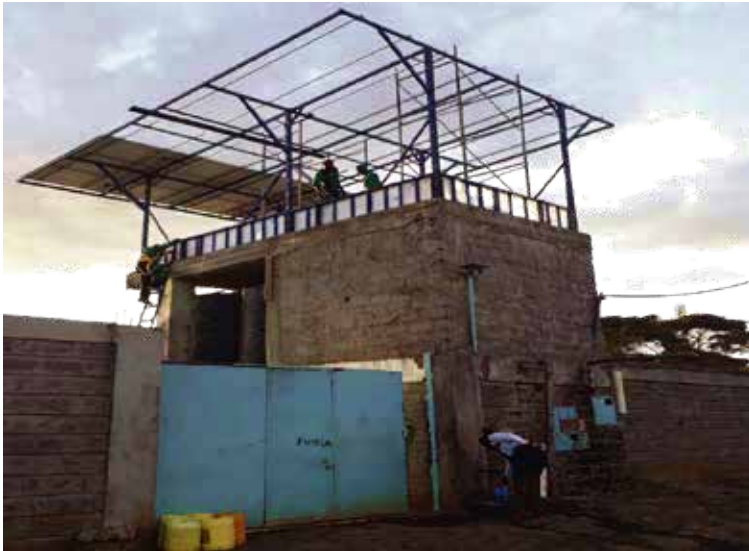
Solar Water Pumping CAPACITY: 11KW Kabiria
